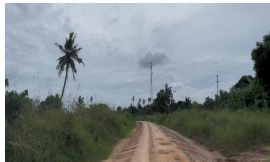
On the right - existing 33kV Distribution line
