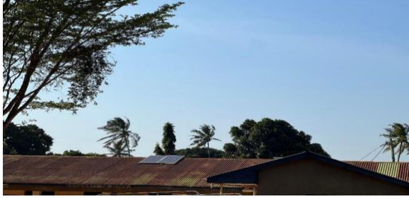
House installed with solar panels
