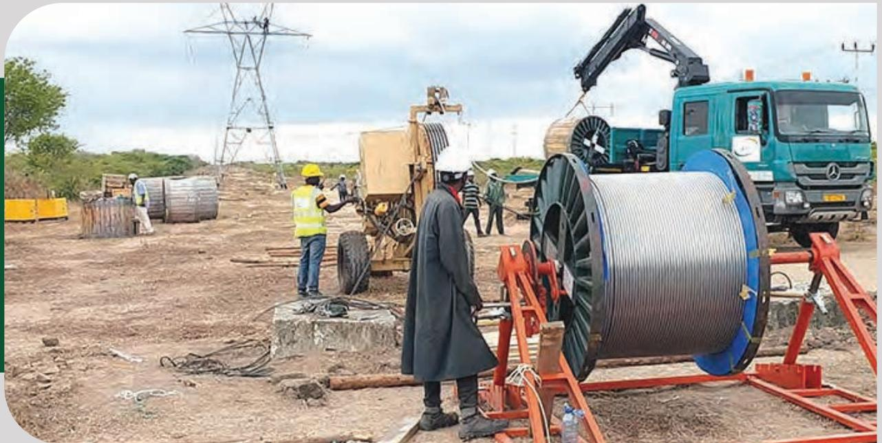
*Preparation and rolling of conductors during the replacement of old ones.*
